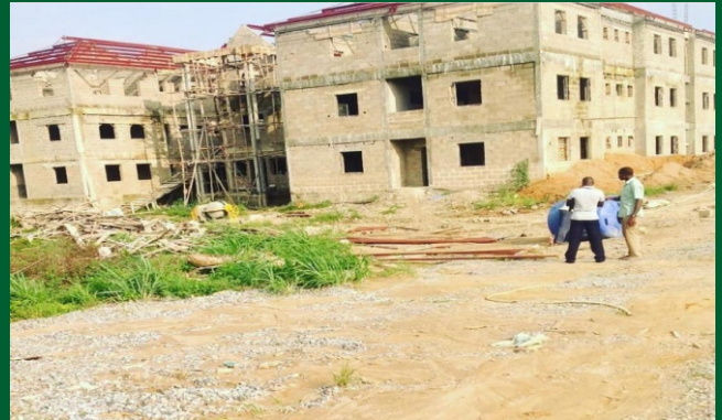
Truss Job at Deeper Life, Mowe
